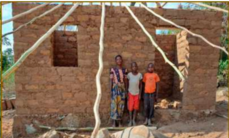
MS with her sons and their nearly completed home
